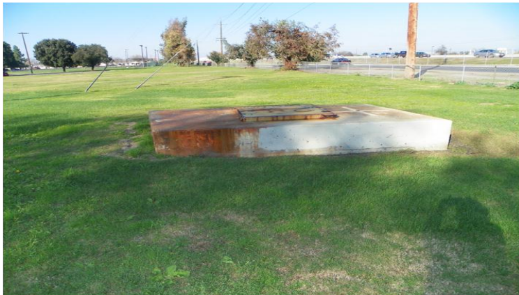
A utility vault at Van Buskirk Park with a cyclone fence in the background. Both show signs of corrosion.
