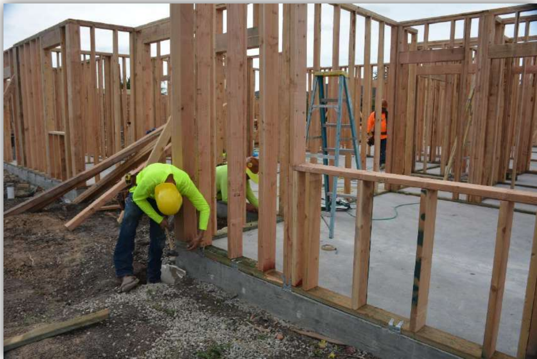
Framing Sierra Vista Housing
