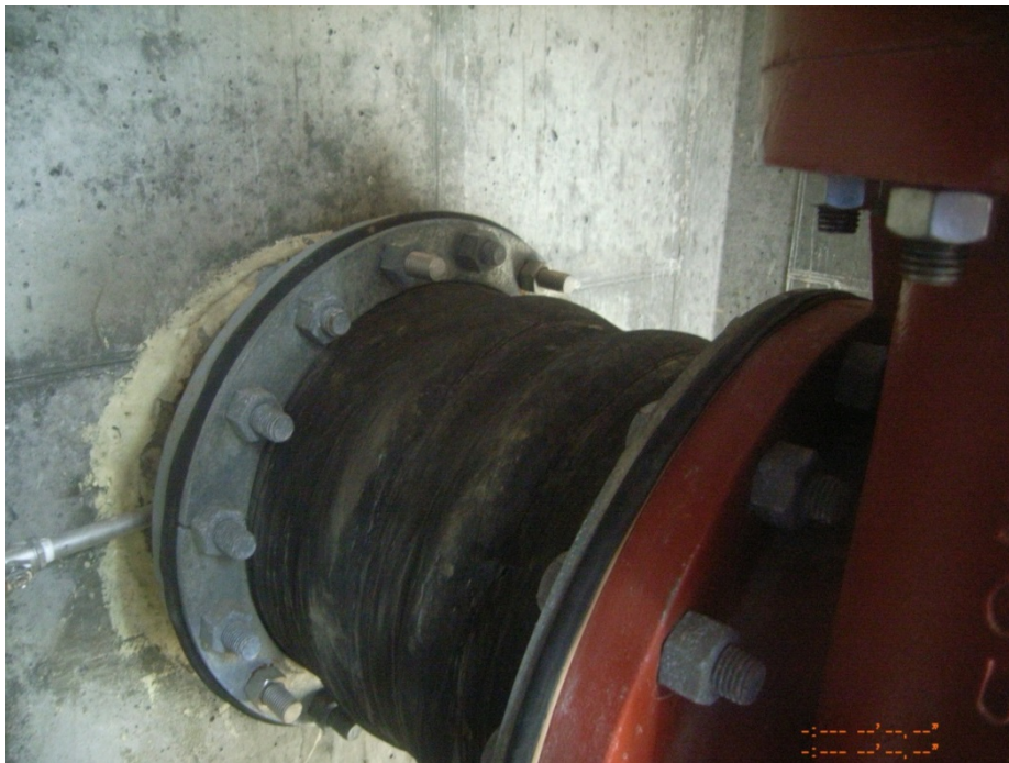
Figure 20. 16-inch pipe connection
