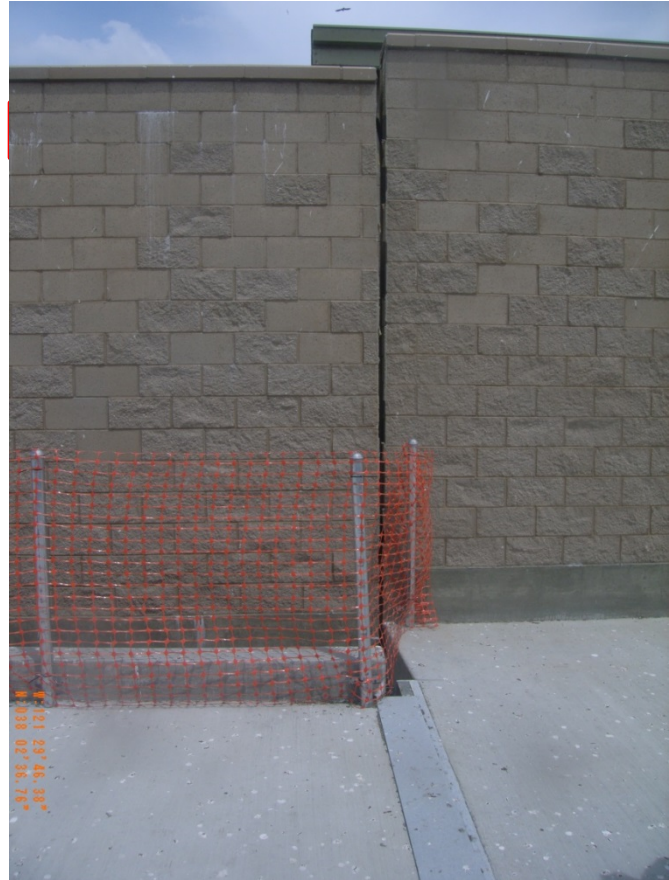
Figure 9. CMU wall displacement located at the south
