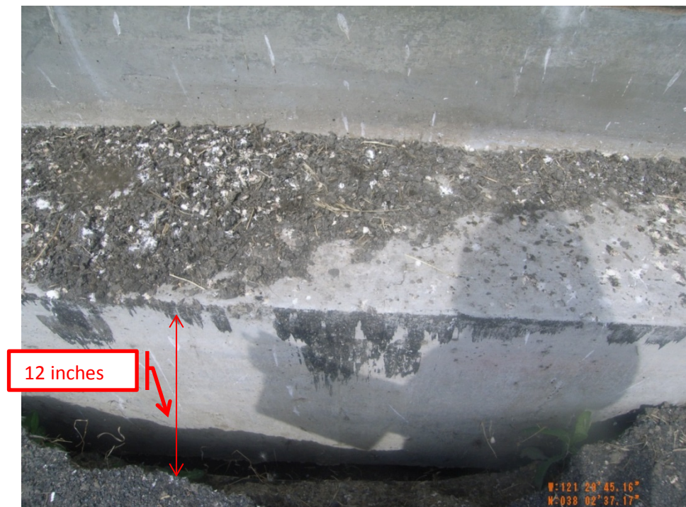
Figure 6. Gaps created between building foundation and surrounding surface (measurement is representative and not a complete survey)
