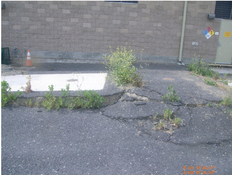
Figure 12. Uneven pavement along north of building
