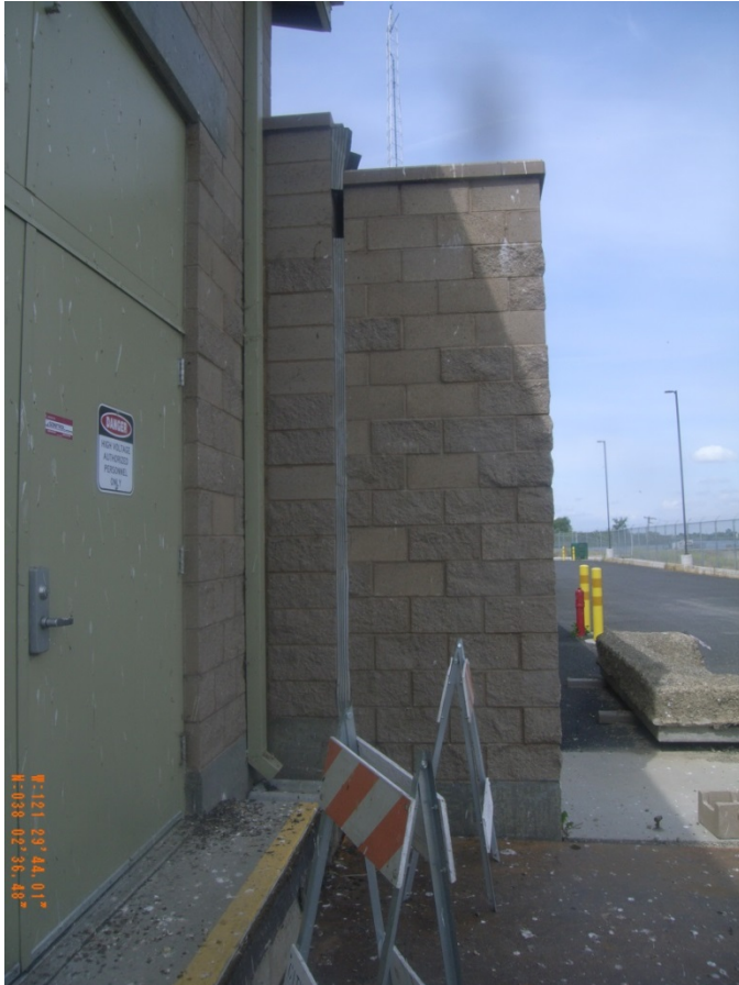
Figure 8. CMU wall displacement located at the north (measurement is representative of the area and not a complete survey)
