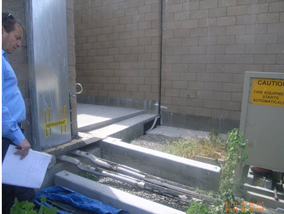
Figure 16. Yard construction repairs - covering plate was removed to allow conduit realignment, various bends were added to the conduit to adjust conduits at the settling ground and pile supported facility; conduits have been left exposed in case of future construction
