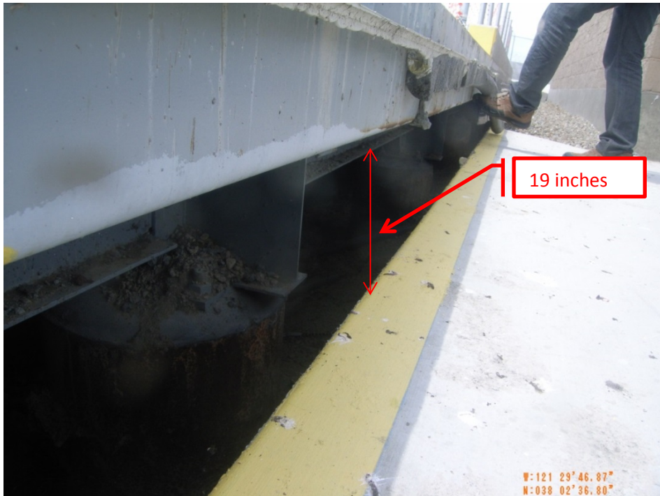
Figure 11. Representative voids along south of building (measurement is representative and not a complete survey)
