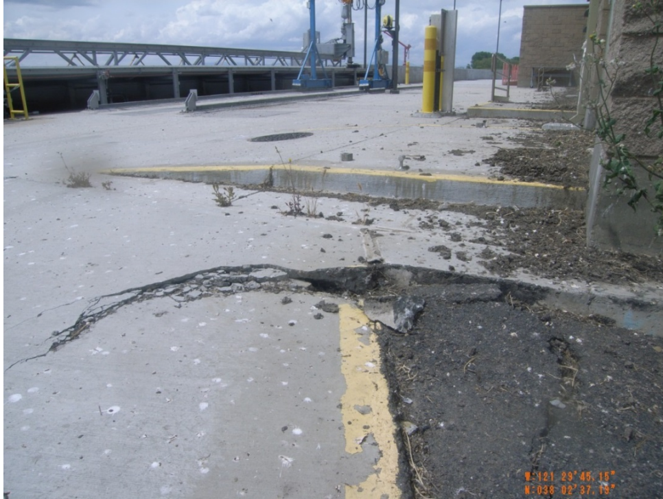
Figure 13. Crack created in concrete due to displacement, south of building
