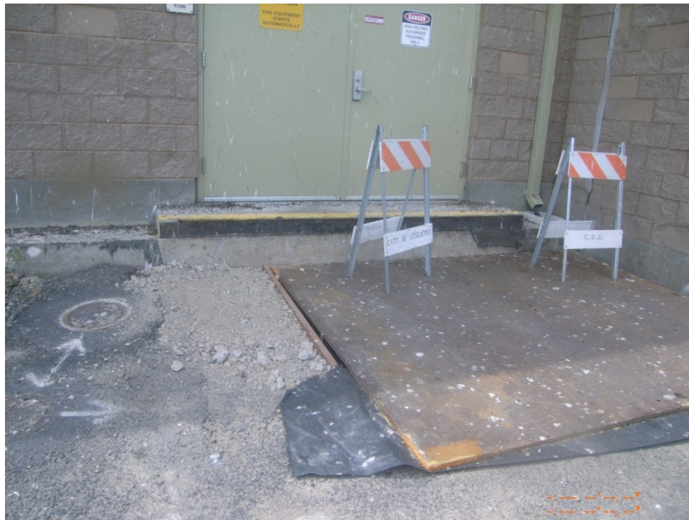
Figure 15. Location of where the building landing was removed to allow for conduit slack to be extended at north side of building
