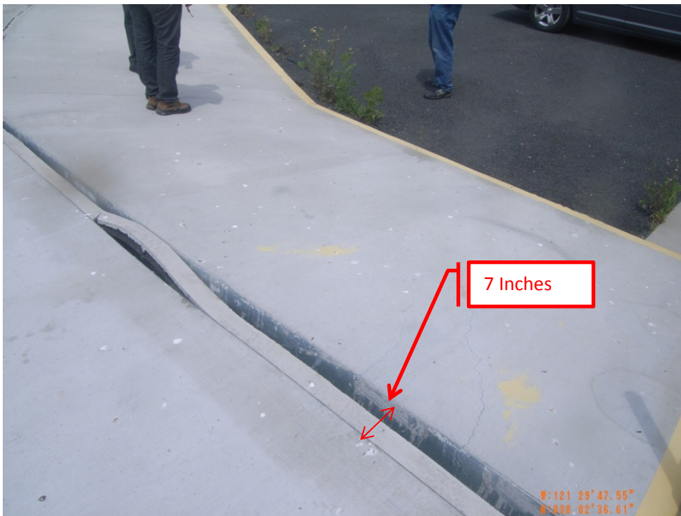
Figure 5. Driveway concrete slab gap (measurement is representative and not a complete survey)
