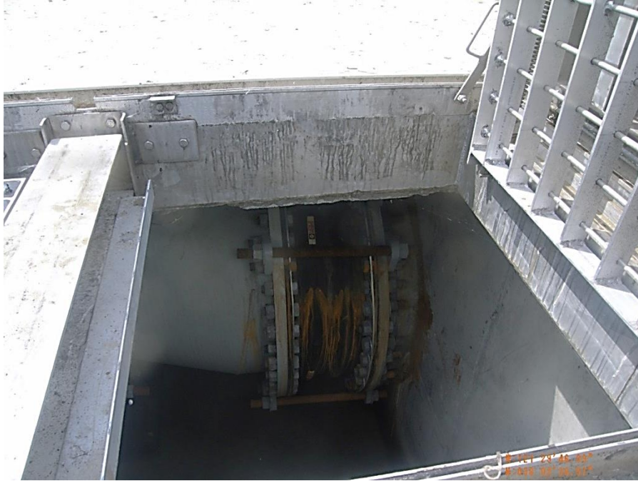
Figure 19. 54-inch double expansion joint pipe connection
