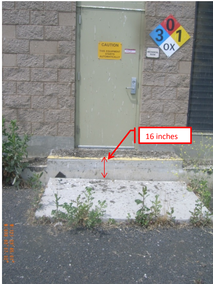
Figure 7. Representative raised doorway step and separation from landing, east entrance door (measurement is representative and not a complete survey)
