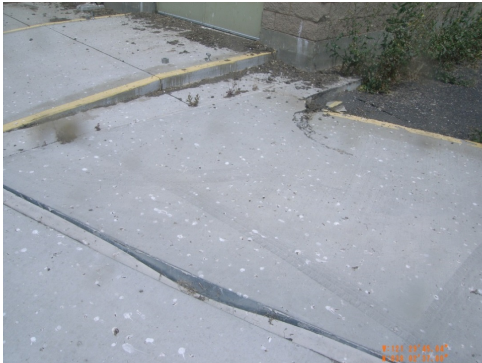
Figure 14. Disconnections in the concrete, south of building
