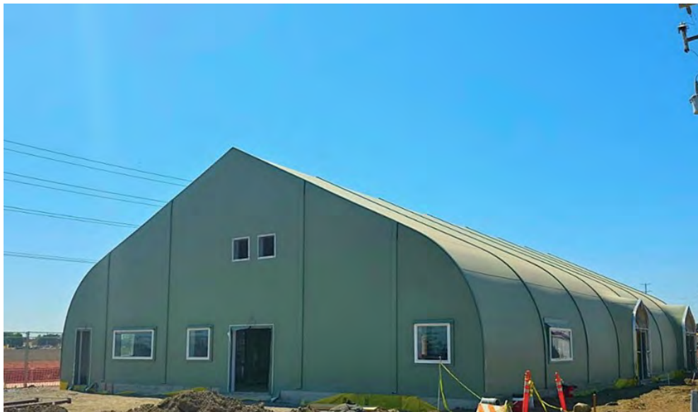
Tracy Shelter Sprung Structure adding 70 beds + congregate room (Photo by: Civil Grand Jury)
