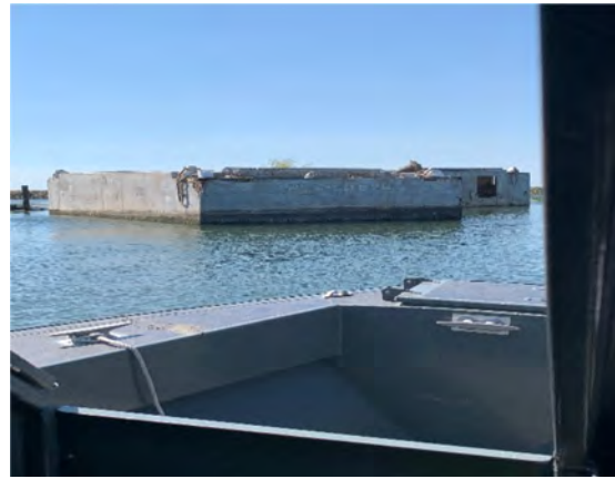
Concrete Structure (Photo by: SJ Sheriff's Office)
