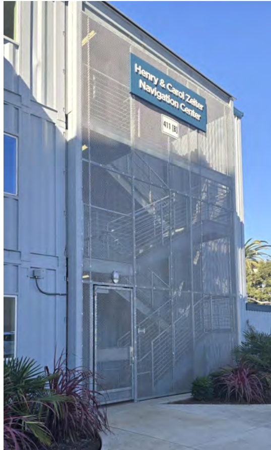
Photo 8: St. Mary's Navigation Center Entrance (by Civil Grand Jury)
