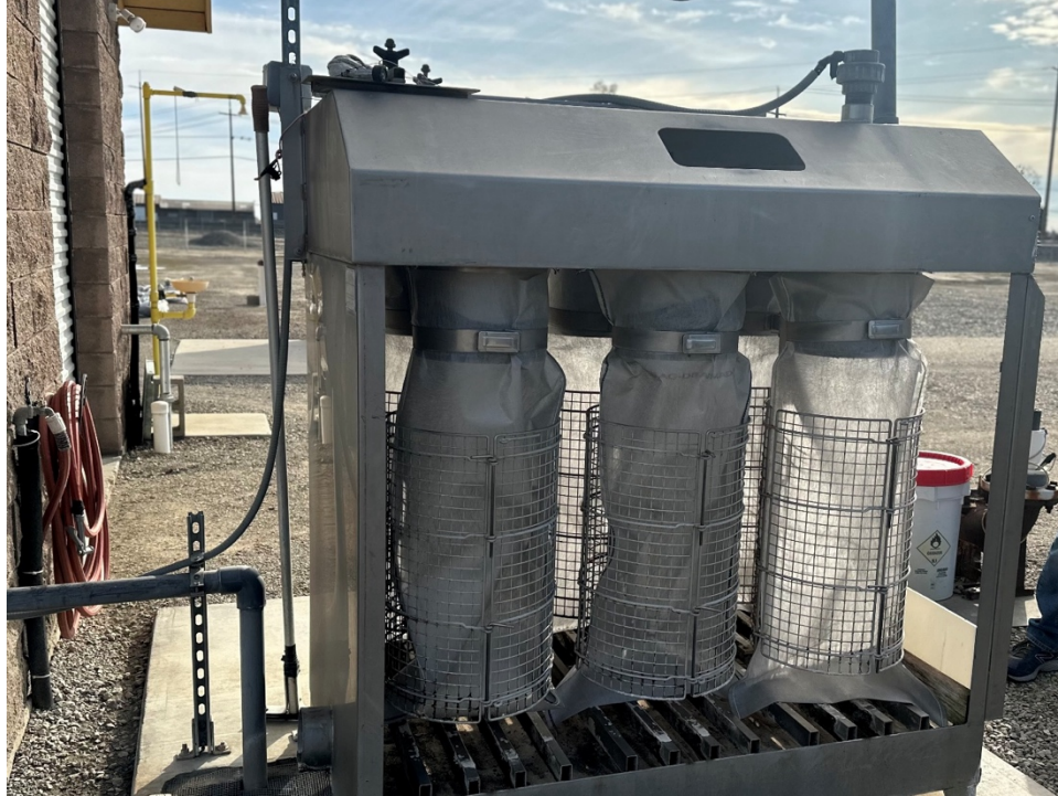
Taken February 21, 2025, bagging stations for bio-solids draining
