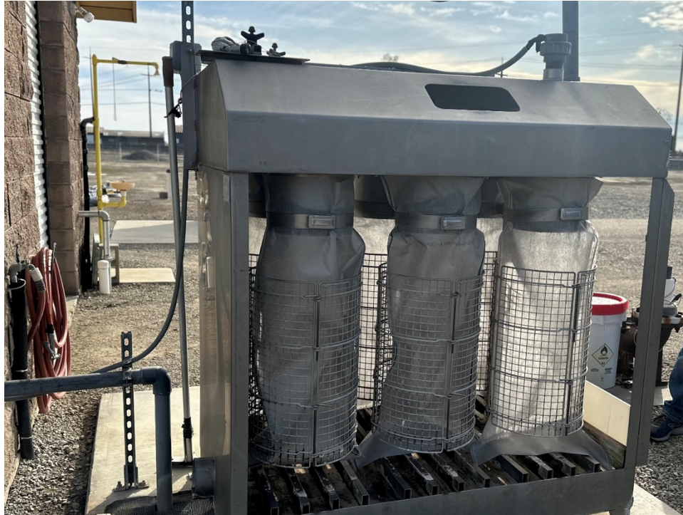
Taken February 21, 2025, bagging stations for bio-solids draining
